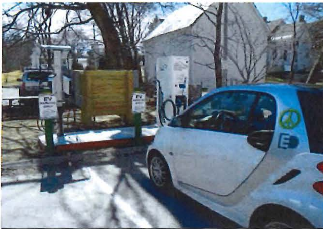
The Town of Bennington has installed several new high-speed electric vehicle charging stations in municipal parking lots in the downtown area.
